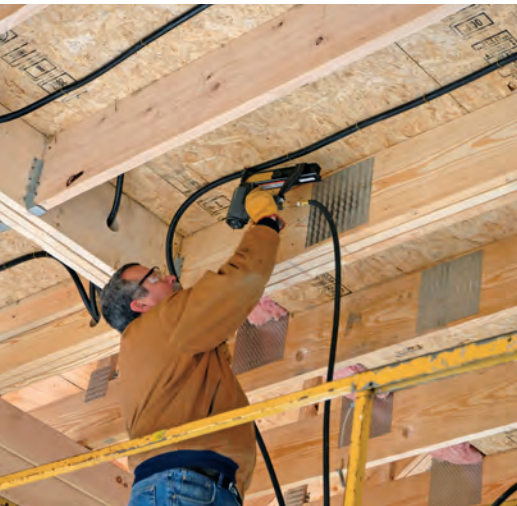
Left: Dave Yates installs hydronic radiant tubes to the underside of the garage subfloor.
