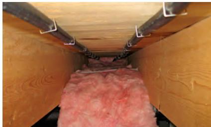
Left: Dave Yates installs hydronic radiant tubes to the underside of the garage subfloor.
