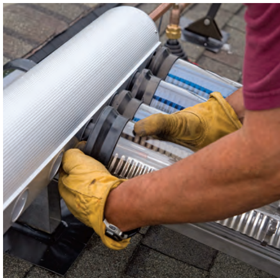
Inserting the evacuated tubes into the header.
