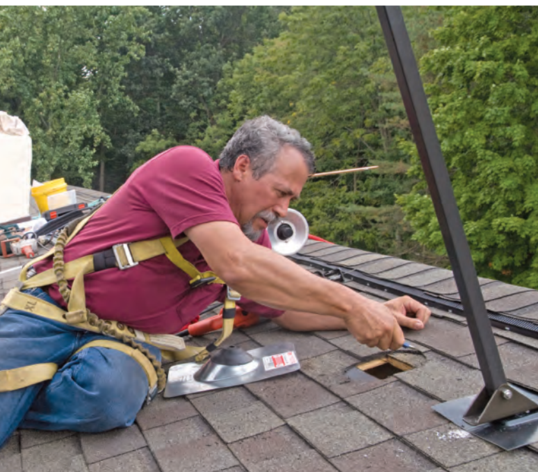
Yates makes the roof penetrations for the thermal lines.
