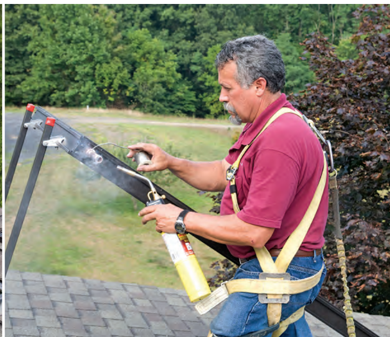
The sweating of the thermal line-sets begins.
